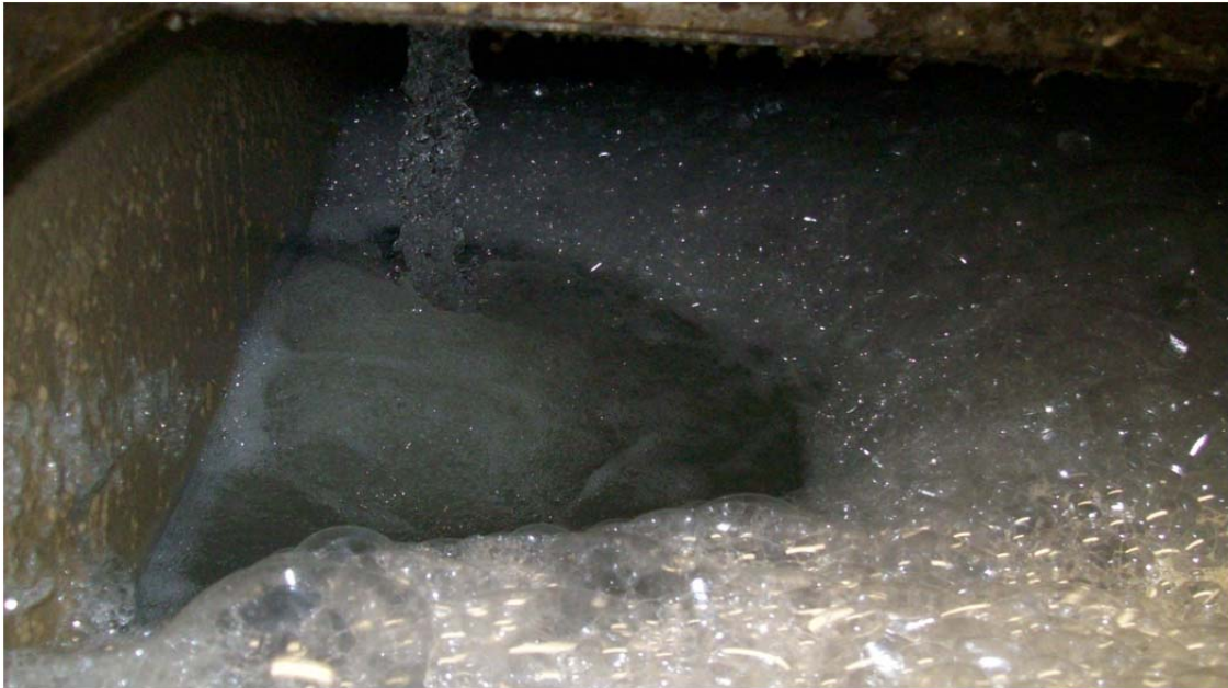
Figure 6: Water Foaming before Ozone treatment (note the organic accumulation on the wall)
